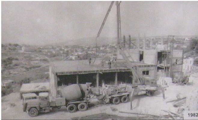
Beginning construction of the high school
