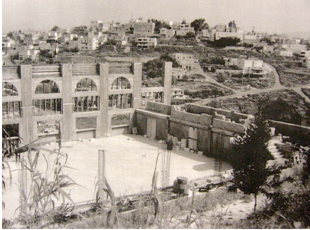
Construction halted on the gymnasium
